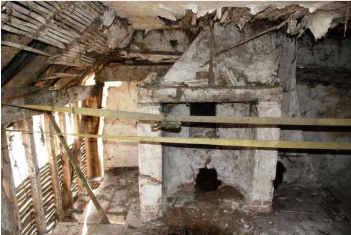
Plate 5. First Floor (looking east)
