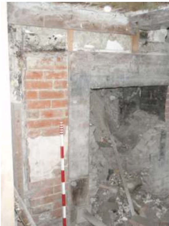
Plate 10. Ground Floor – close up fireplace
