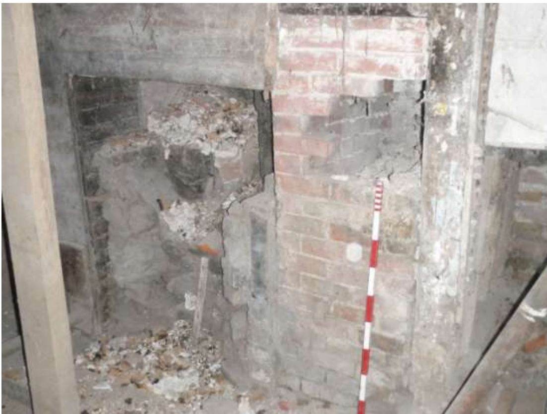
Plate 8. Ground Floor – close up fireplace
