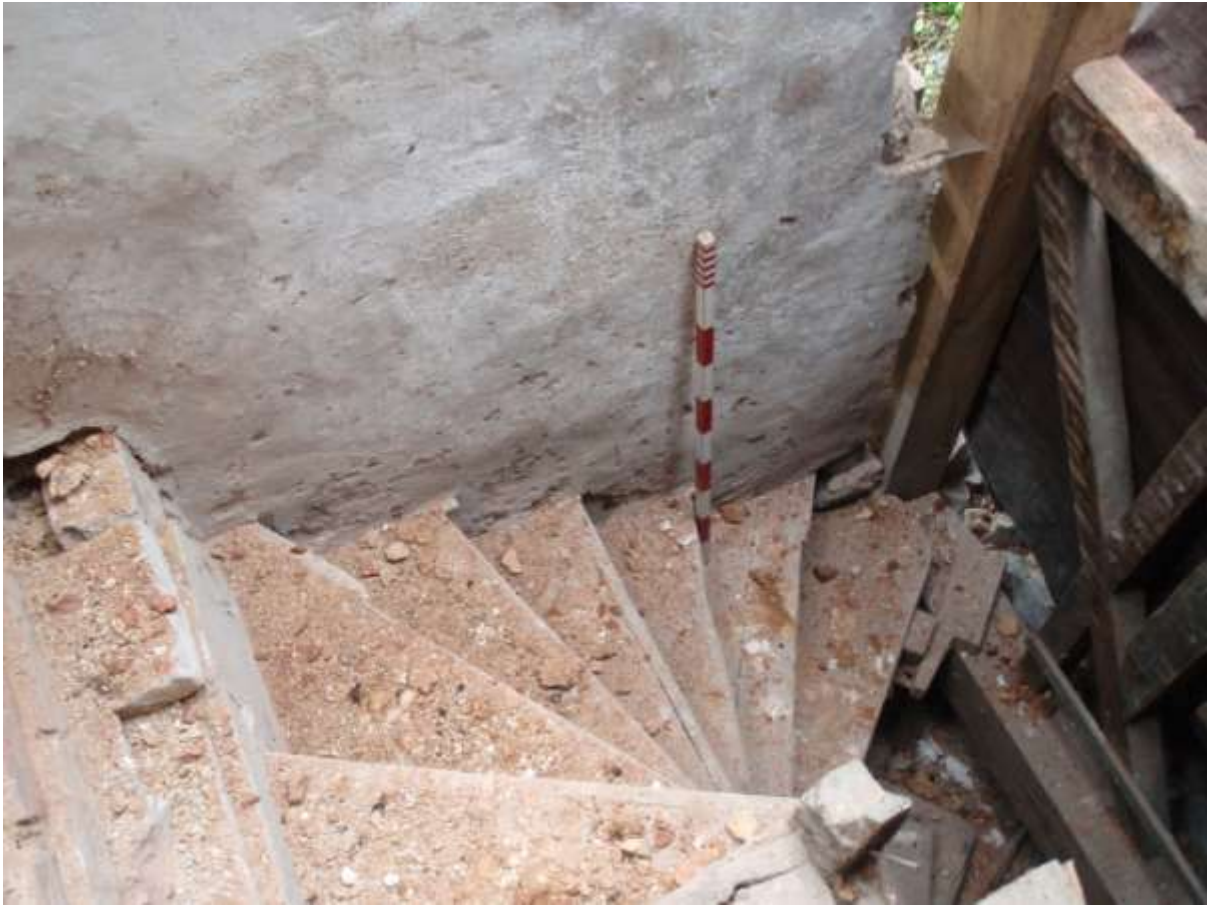
Plate 13. Stairs to the right of chimney
