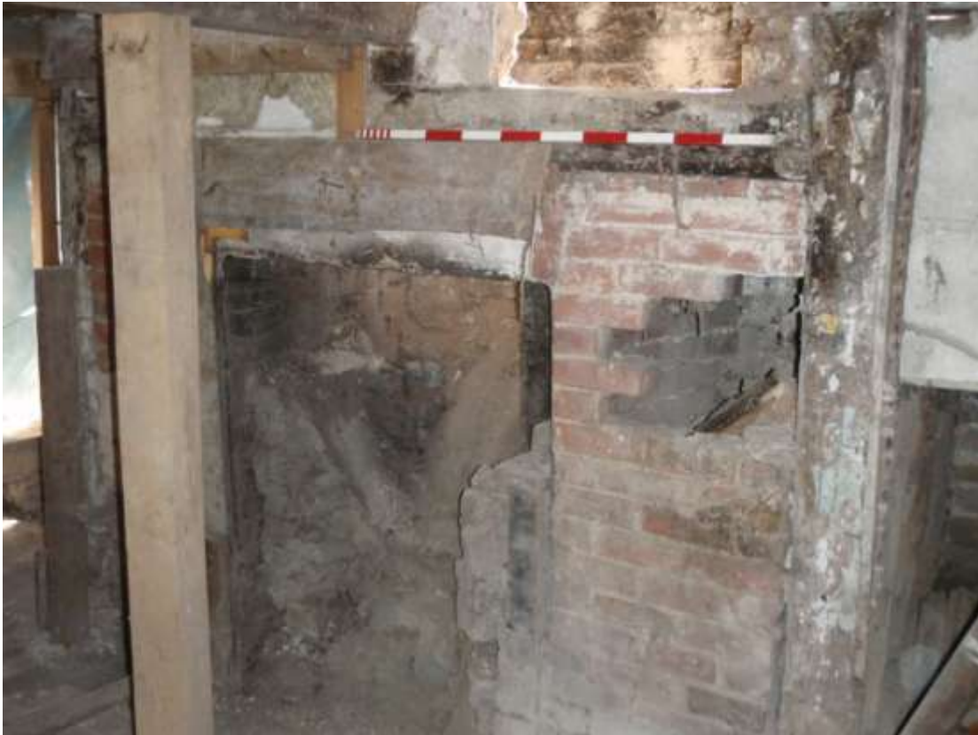
Plate 7. Ground Floor – close up fireplace
