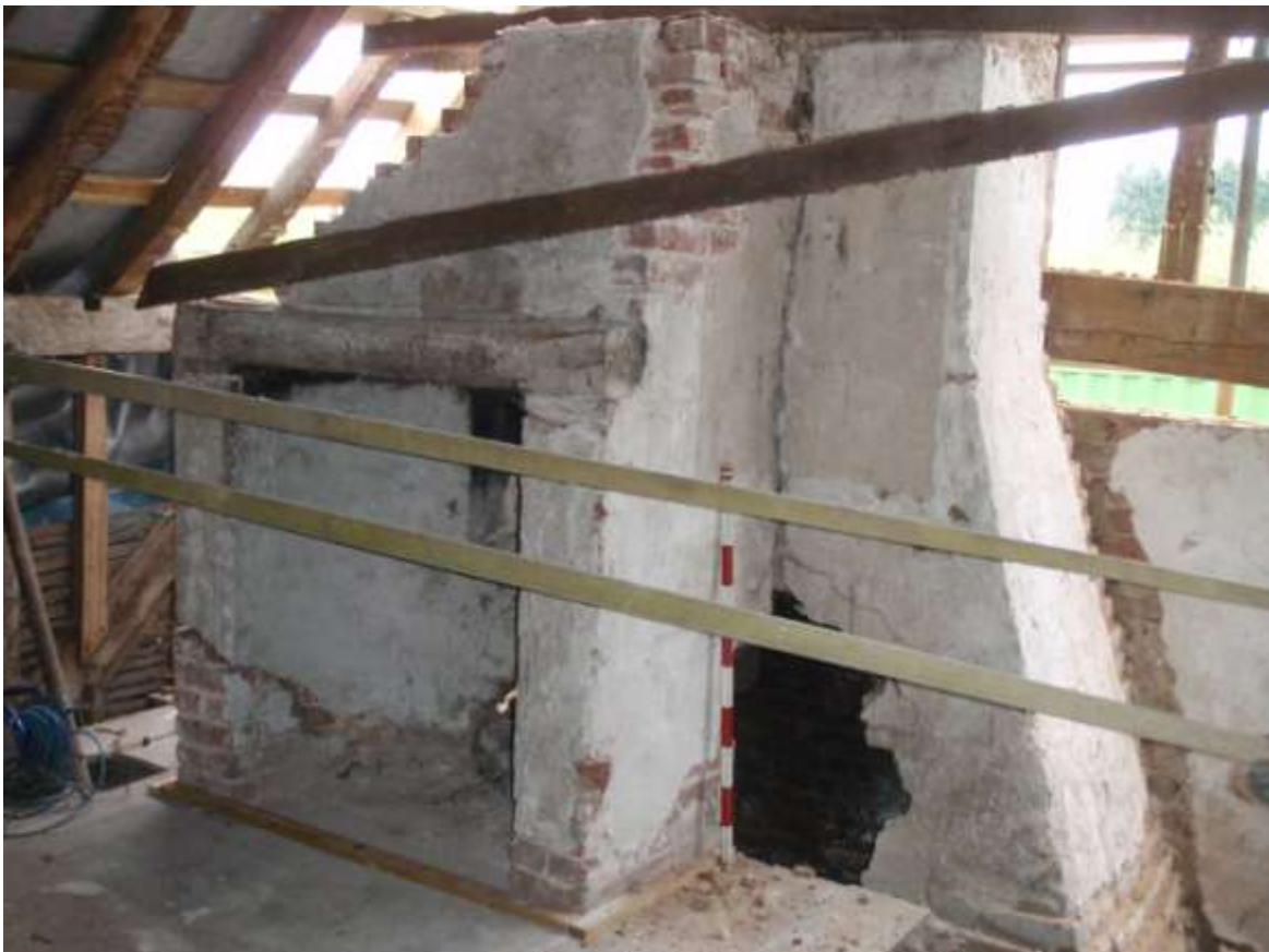
Plate 6. First Floor (looking NNE)
