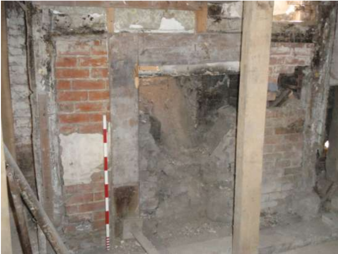
Plate 9. Ground Floor – close up fireplace
